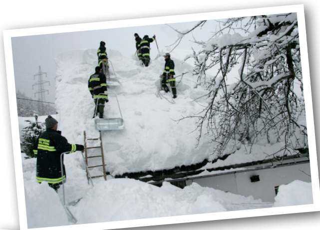
After heavy snowfalls roofs have to be freed from snow to avoid damage.
